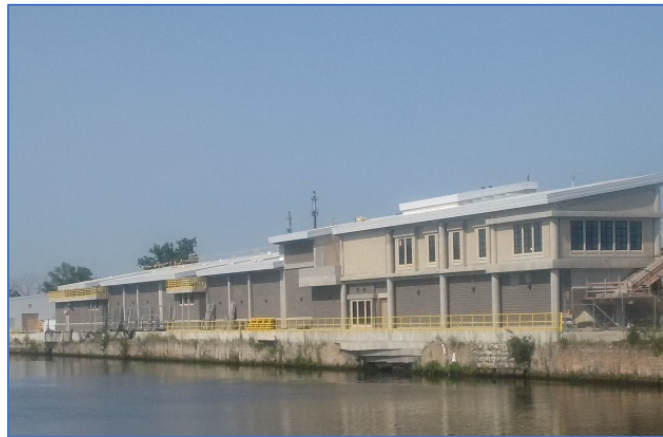
Permanent Barrier I. Photo Credit: USACE
